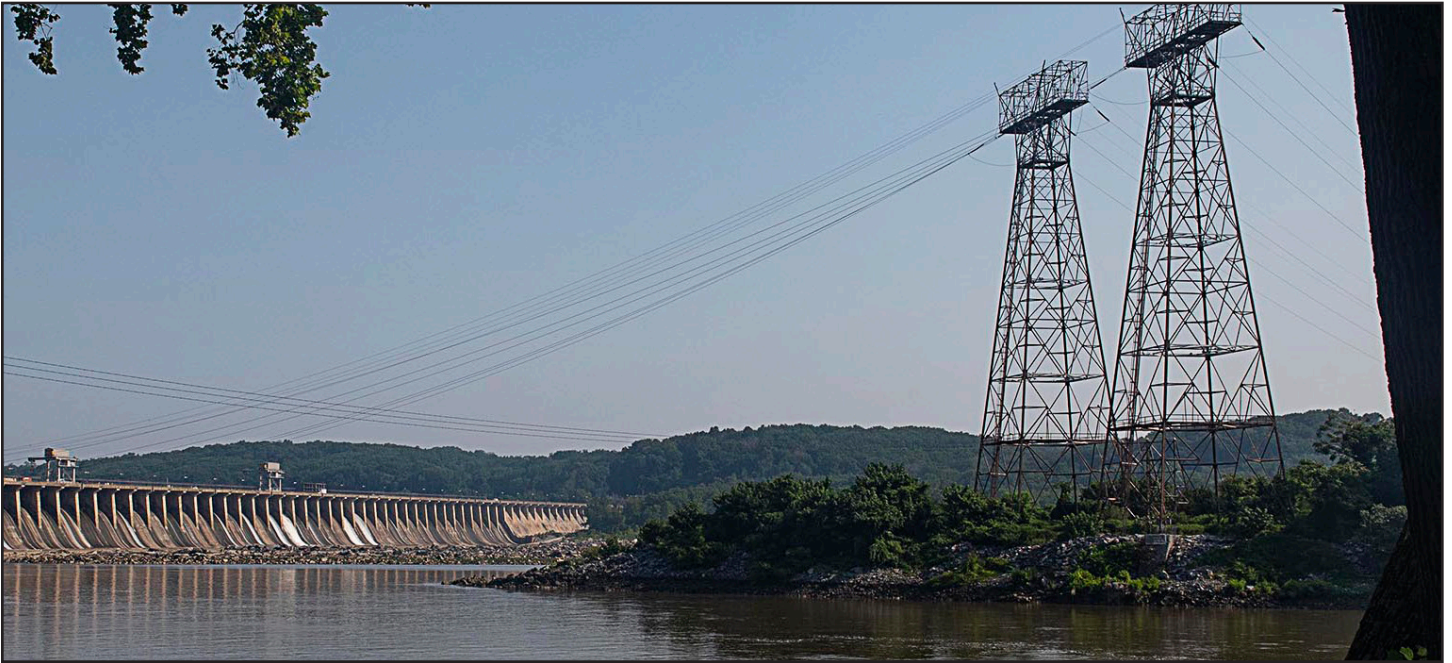
Photo Courtesy of Conowingo Dam, Tony DeYoung
