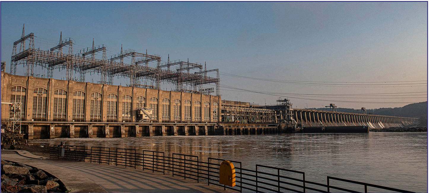
Photo Courtesy of Conowingo Dam, Tony DeYoung
