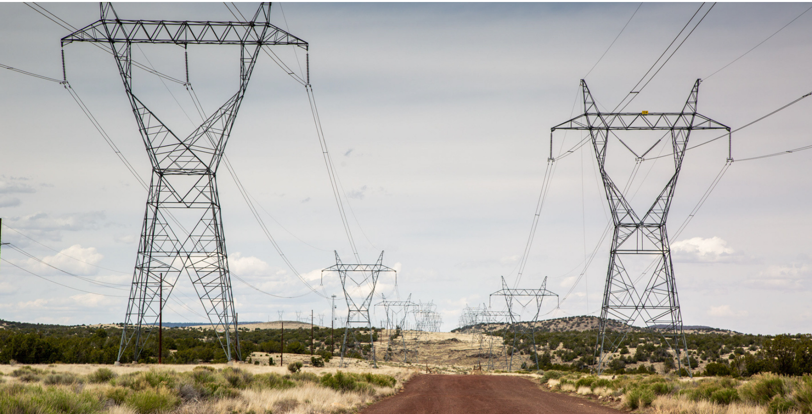
Photo Courtesy of U.S. Department of Energy – Western Area Power Administration
